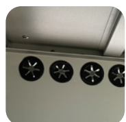
Rubber cable ports.
